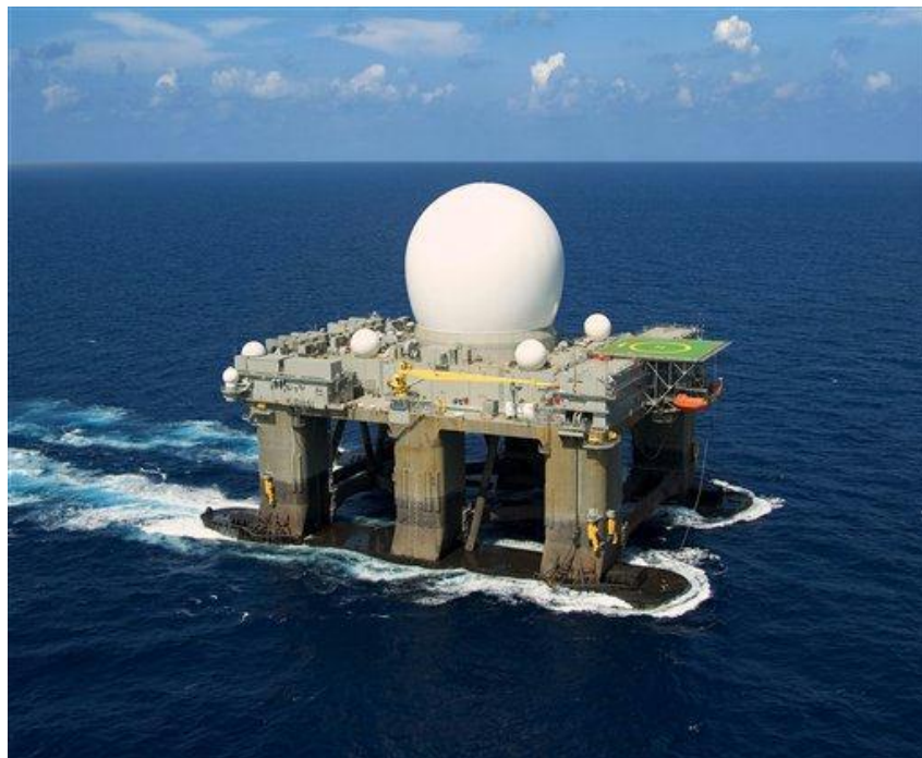
SBX-1 fully afloat and under way
